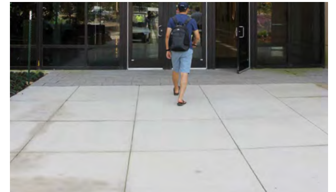
Concrete paving used at building entry plaza
