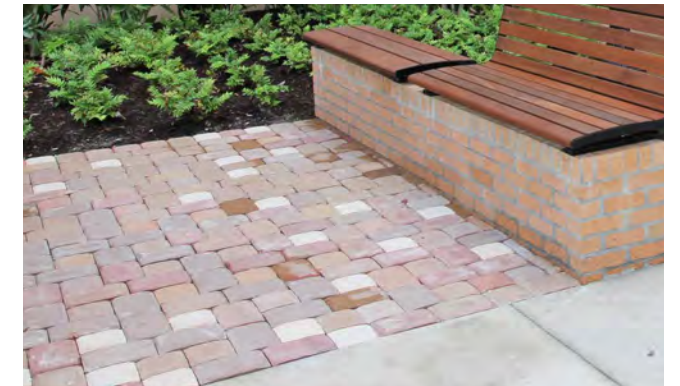
Pavers used to distinguish a seating area
