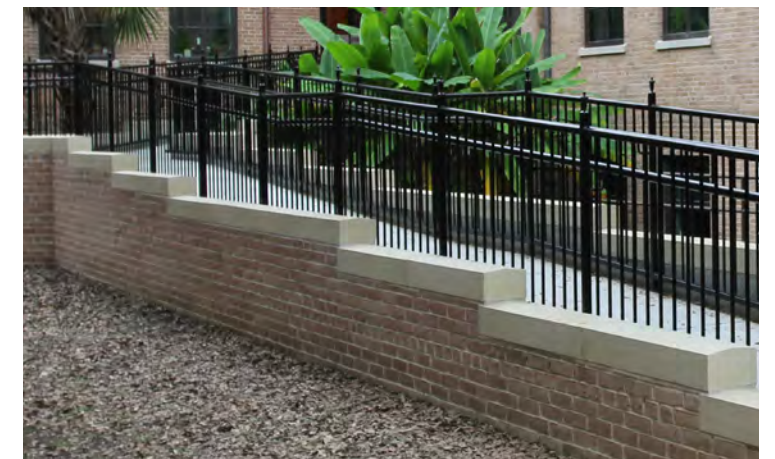
Wooden Hall retrofit ramp avoids existing trees
