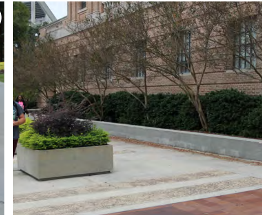
Walls for planting should be used when they can also serve as a form of retaining or seat wall
