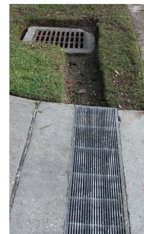
Trench drains at paving edges and supplemented by catch basin
