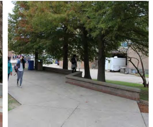
Good combination of retaining and seat walls
