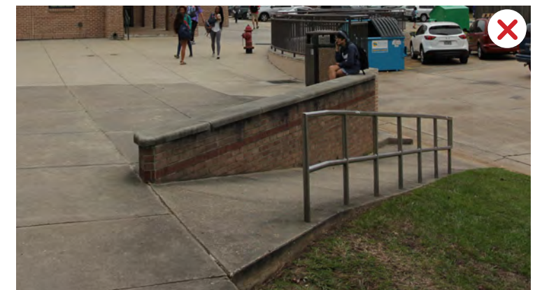
Tureaud Hall ramp lacks the appropriate slope & handrails
