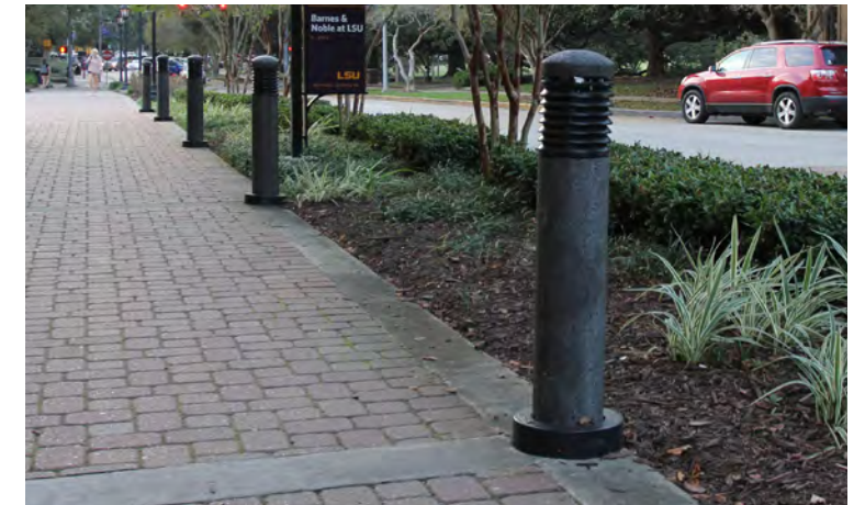
LSU Campus - use of bollards as primary illumination not recommended
