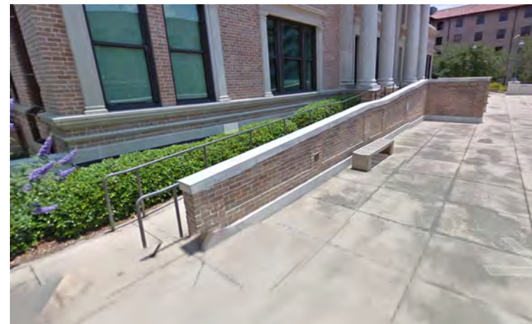
Journalism Building ramp integrated into architecture
