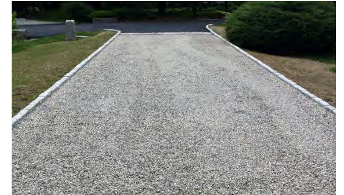
Crushed limestone as a vehicular paving surface
