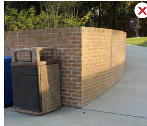
Taller retaining walls over eye level should be avoided
