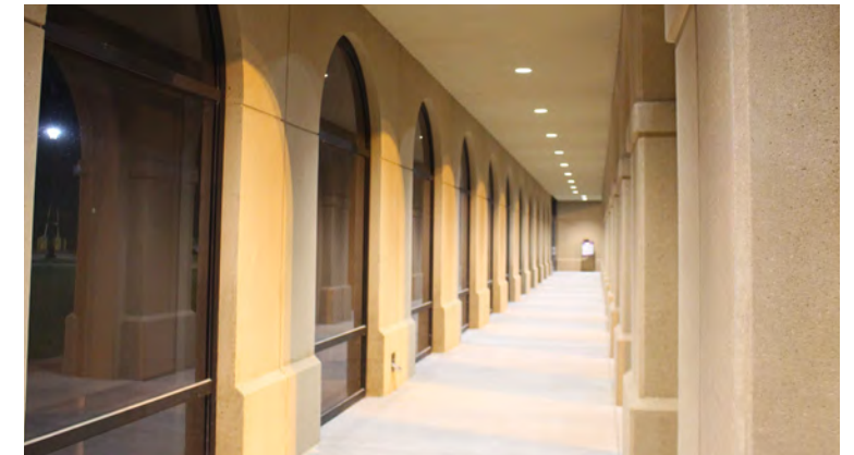
LSU Campus - Example of recessed downlighting along exterior corridor
