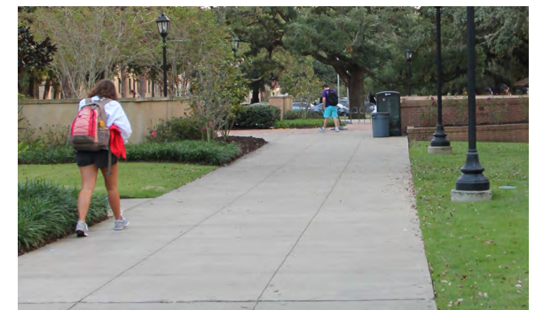
Primary walk with concrete paving
