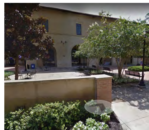
Freestanding wall, appropriately embedded in garden, defines the edge of a plaza space
