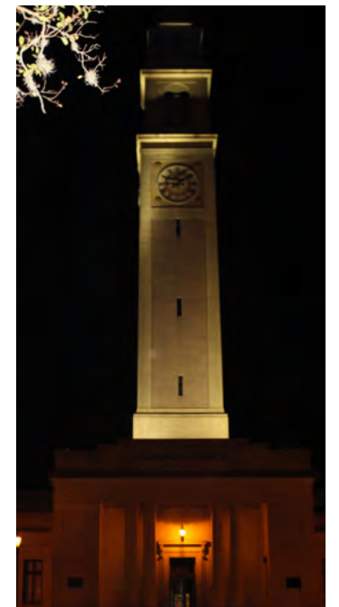
LSU Campus - Example of accent lighting. Lighting effect could be improved by more even illumination of the tower and standardization of color temperature of lighting elements. Tower is a good color while lower level lighting is very orange.
