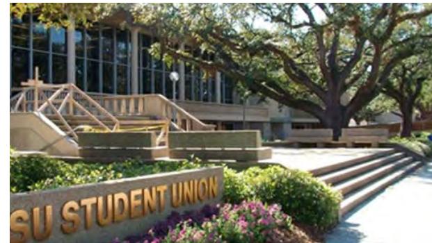
The south stair reaches into the landscape
