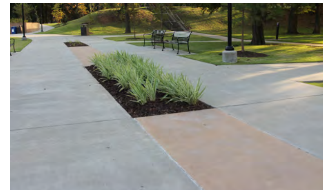
Combined vehicular and pedestrian concrete paving
