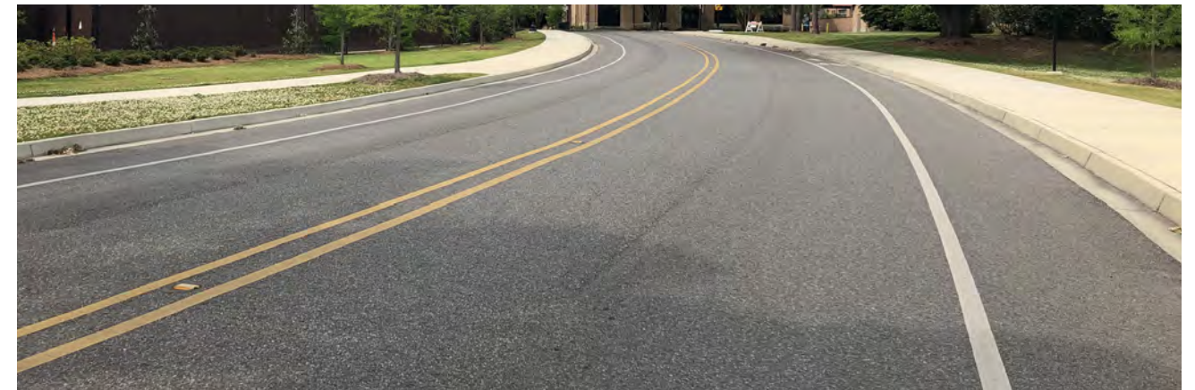
Typical asphalt roadway application on campus
