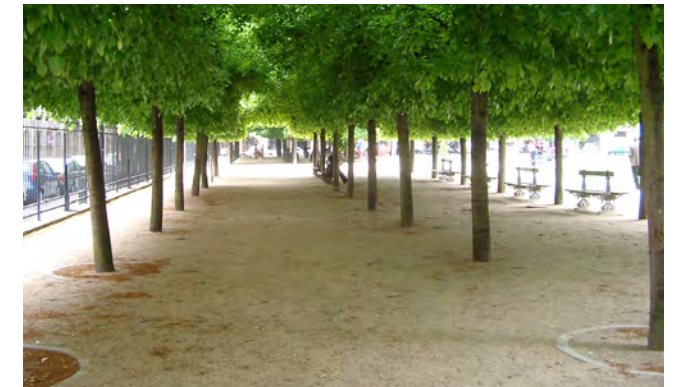
Decomposed granite paving around trees
