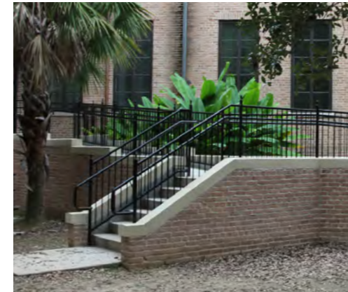
Retrofit stairs with materials matching adj. building
